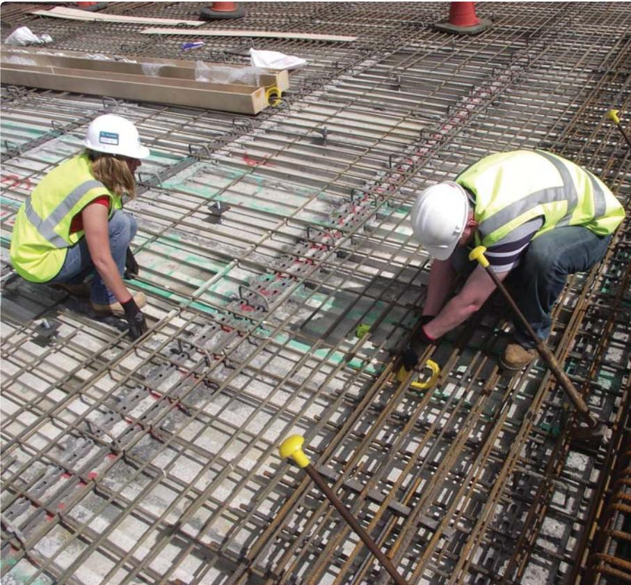
Figure 5: Positioning of BFRP bar with fibre bragg grating sensors.
